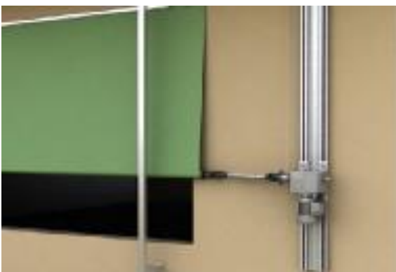
BOTTOM-UP LOCK DRIVE SYSTEM
